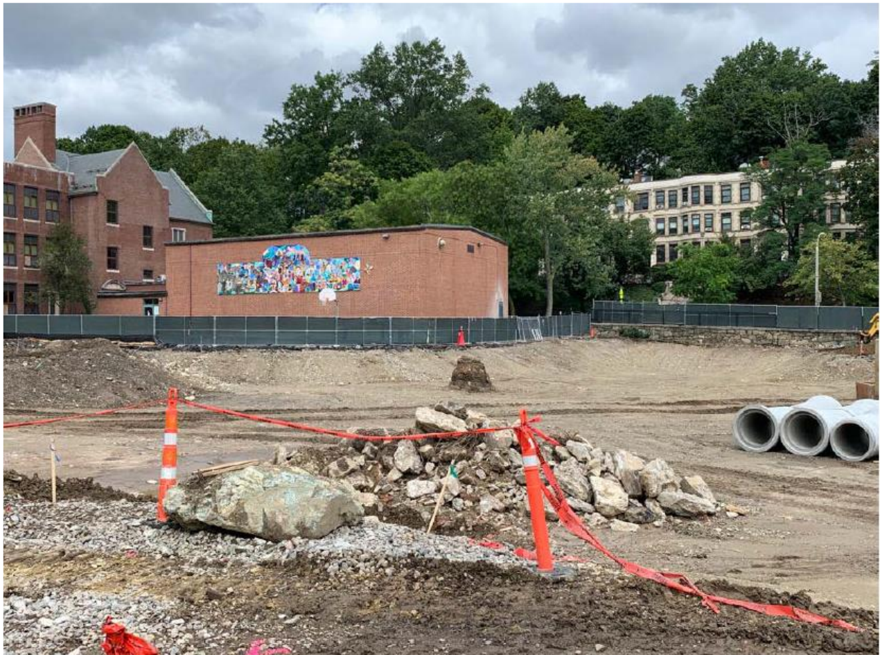
5 Feet of Soil Removed from Site
