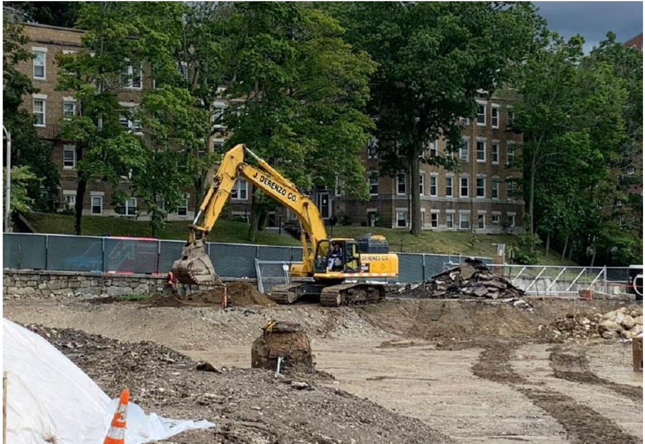
Pre-Trenching Commenced at Westbourne Side of Site
