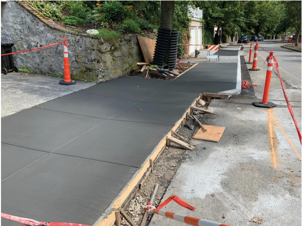
Sidewalk placed along Westbourne Terrace
